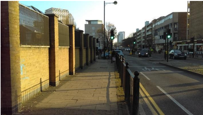
Existing wall and fencing along Roman Road, which would be filled in by green screening inside the school boundary
