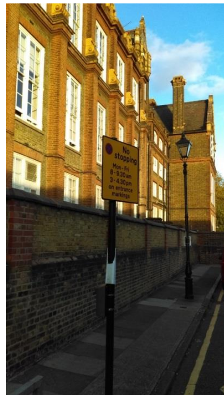
Ropery Street frontage, showing single yellow line stretch of kerbside where waiting is not permitted during the times shown
