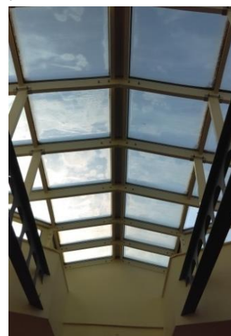
Central skylight (Bethnal Green)
