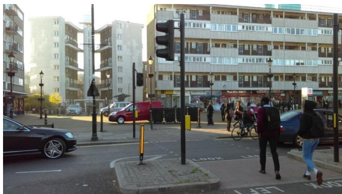
Roman Road signalised intersection, showing pedestrian crossing facilities and wide footways
