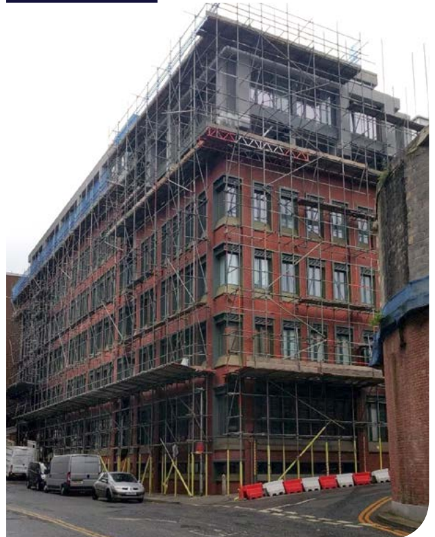
The appearance of Garrard House on the site visit
