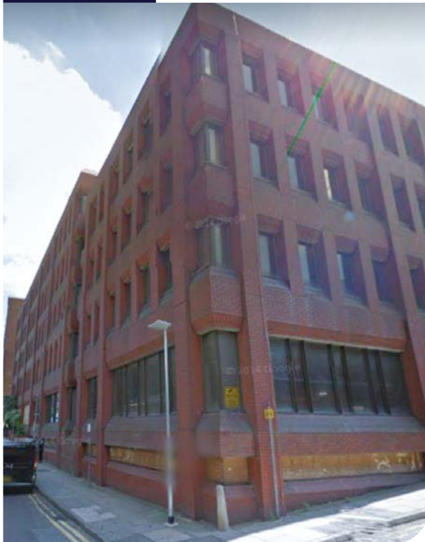
Historic view of Garrard House from 2012
