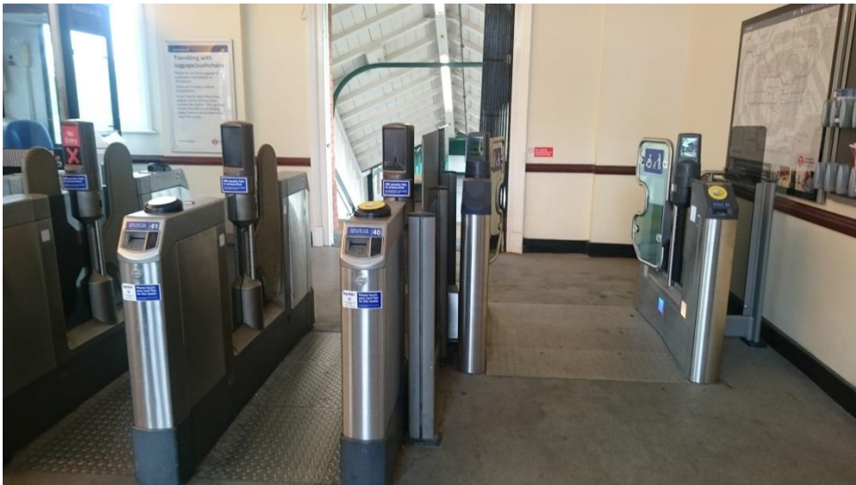
Figure 4 - Gateline left open at Buckhurst Hill, 26th October 2016
