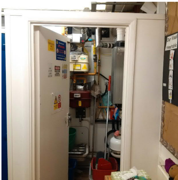
Boiler room and storage cupboard ventilating into classroom
