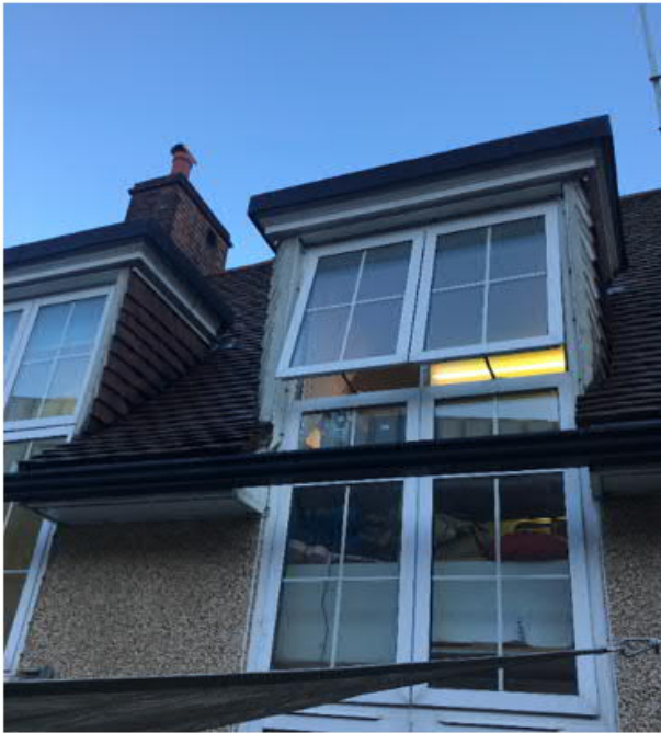
Building reliant on natural ventilation
