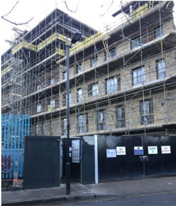
Peckham Place development under construction immediately opposite the nursery.
