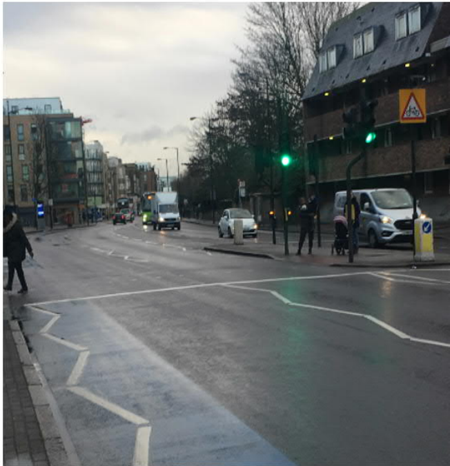
Pedestrians crossing 4 lanes of traffic to reach the nursery.
