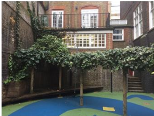
View from the playground of the smaller building on the corner of Laystall Street and Rosebery Avenue (containing the IT suite and other rooms)
