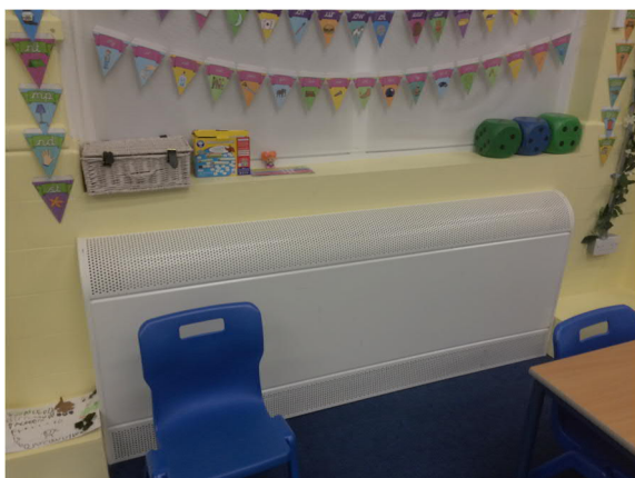
Example of covered radiator in a typical classroom. Teachers do not have control over the temperature of these radiators.
