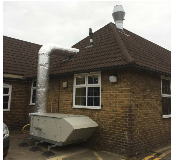
Air intake equipment from the new kitchen
