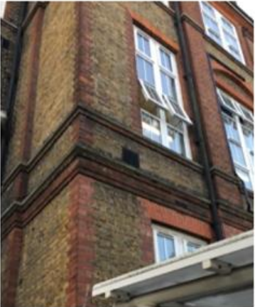
Natural ventilation onto Stanton Way
