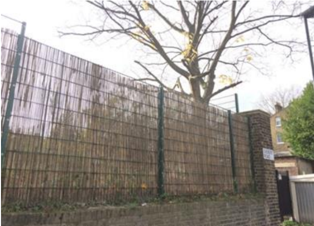
Siebert Road - bamboo fencing on the north boundary of the school site (next to the nursery/reception playground & garden)
