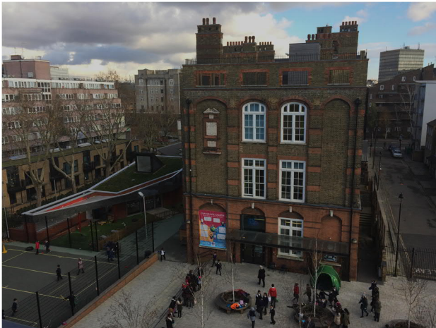
The old Victorian Building viewed from the roof of the new building, with the Acorn Centre to the left
