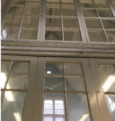
Main Building Windows
