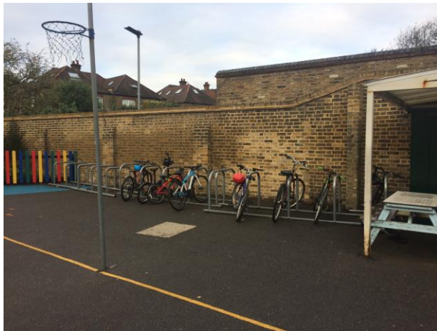
There is lots of cycle parking on site, though it is not protected from the weather
