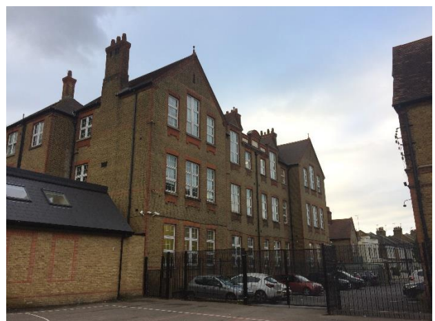
The main school building, viewed from the Key Stage 2 playground. Most of the classrooms are on this side
