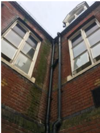
Some classrooms reliant on natural ventilation
