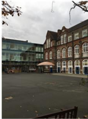
New extension adjoining original building
