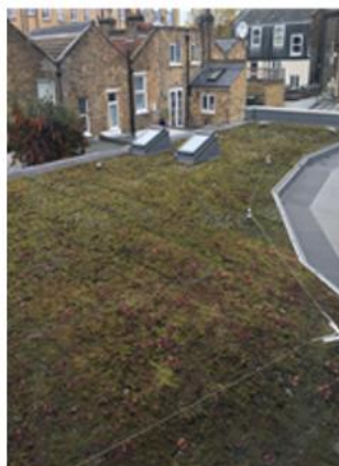
Sedum roof on early years/ nursery classrooms
