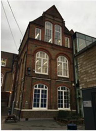
Original school building reliant on natural ventilation
