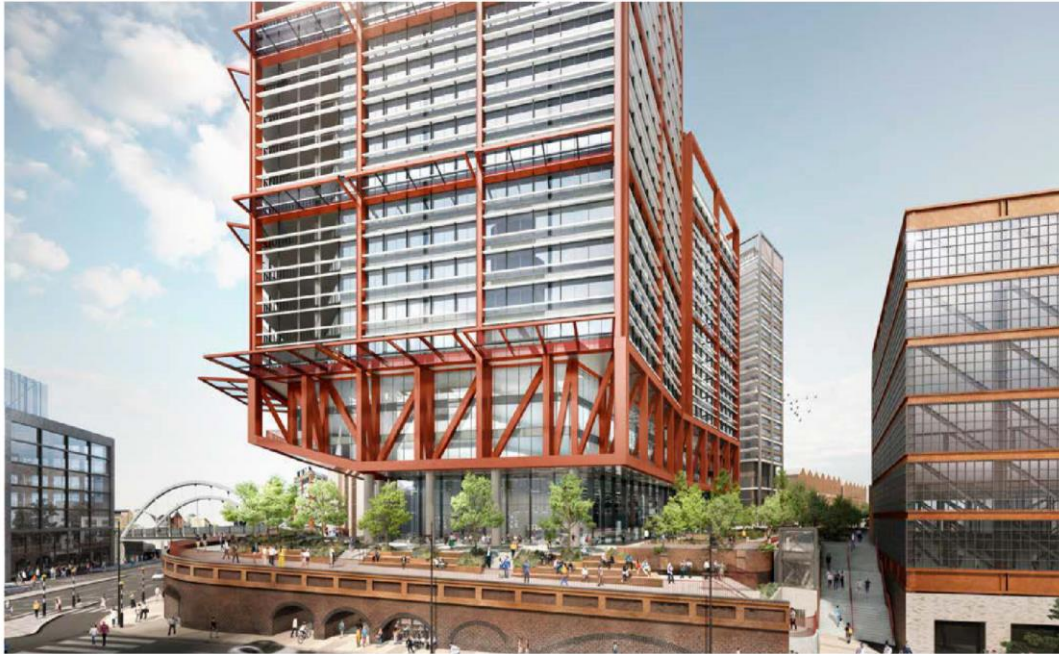
Figure 26: image of the lower floors of Building 2 showing the cantilevered prow and wind mitigation fins
