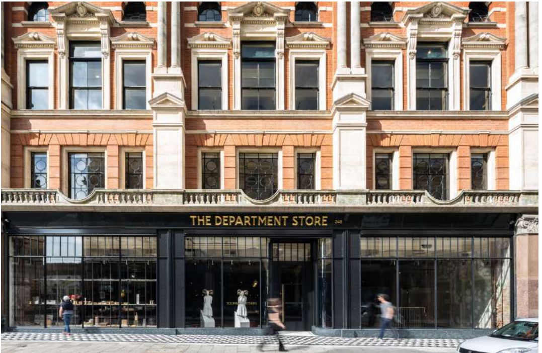
The Department Store, in London, is a landmark Edwardian department store which has been refurbished and reimagined to house workspace, retail units, a cafe, large event space, post office, restaurant and bar. Image credit: The Department Store
