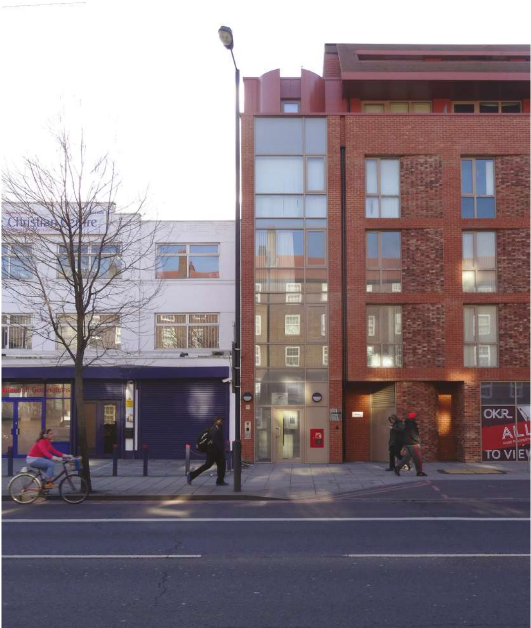
Old Kent Road, LB Southwark
