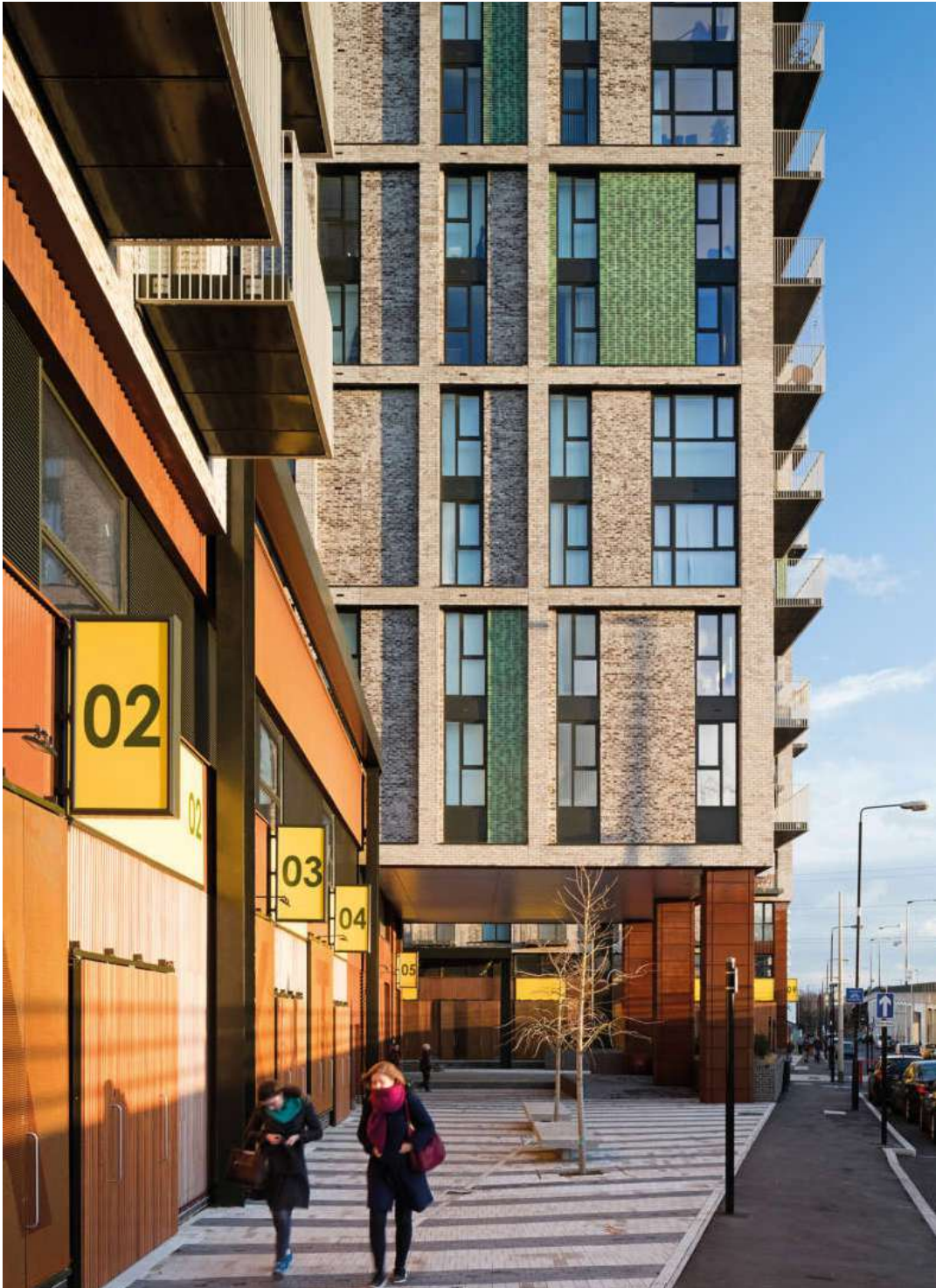
Caxton Works, in London, combines light industrial units at ground floor level with residential above demonstrating the potential for forward thinking and bold mixed-use typologies in the capital. Image credit: Studio Egret West
