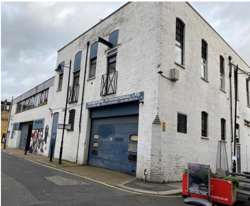
Figure 2 – the existing warehouse at Nos 1-7 and 9 Fenning Street
