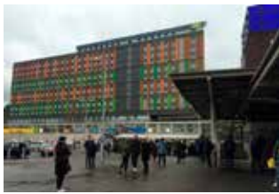
Tottenham Hale Station
