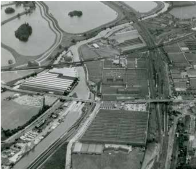
Aerial view of Hale Wharf Site and Harris Lebus Works Looking South 1960s © www.harrislebus.com
