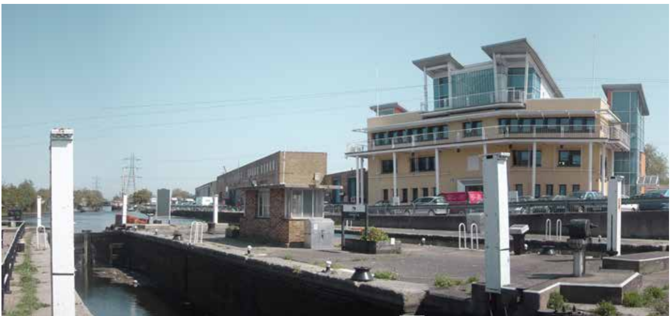
View from Ferry Lane towards River Lee Navigation Channel over Tottenham Lock
