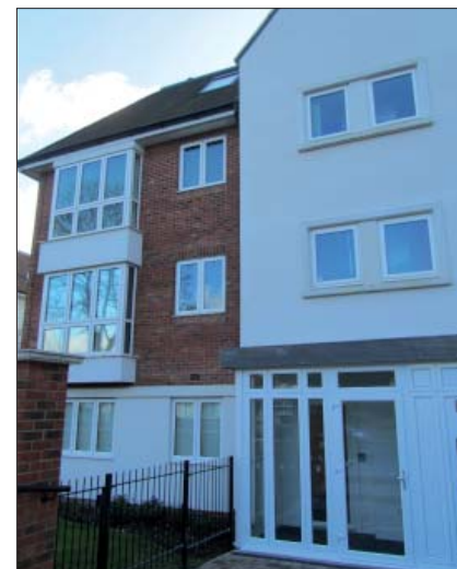
The building fabric remains in very good condition.
