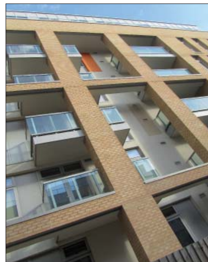
The use of high quality materials is evident across the scheme (except Block A).
