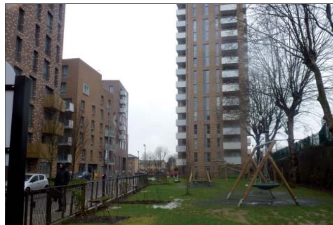
Adjacent blocks within the wider development area are much higher in height.
