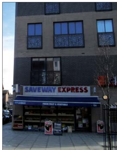
Convenience store to ground floor of development.
