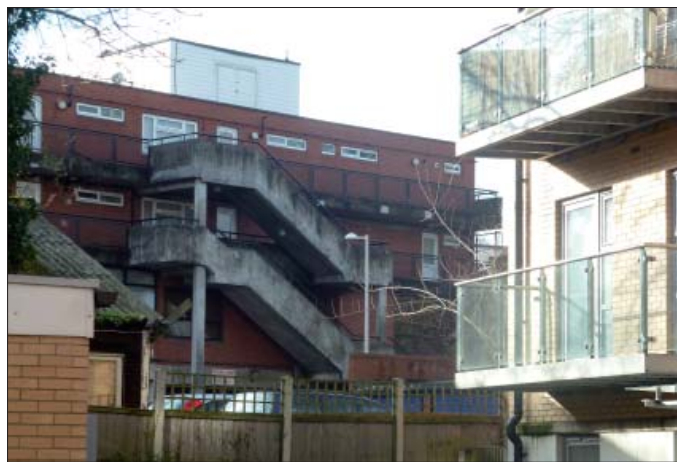
The rear view of the South Woodford Library provides an unattractive outlook to flats within Blocks C and E.
