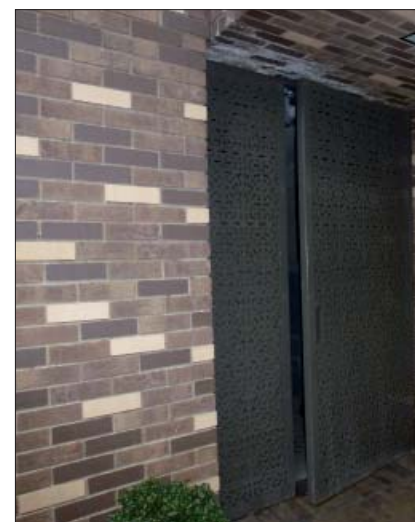
The building fabric has generally performed well since completion.
