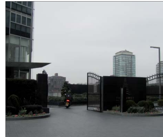
Formal amenity space is provided at the gated entrance to the Tower, with little usable space to sit or relax in.
