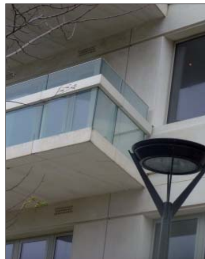
The building fabric has performed very well since completion.
