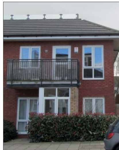
Building fabric has generally performed well since completion.
